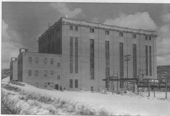
National Research Experimental (NRX) reactor, Chalk River, Canada. (Courtesy of AECL)
