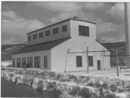
Zero Energy Experimental Pile (ZEEP), Chalk River, Canada. (Courtesy of AECL)
