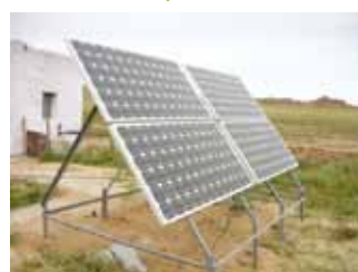
Improved installation with wind-control
